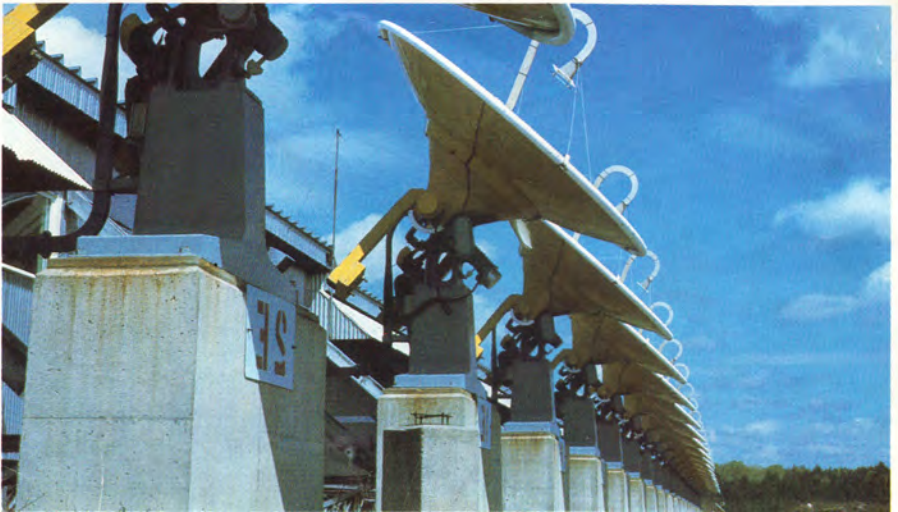
The solar array is composed of 32 dishes.
